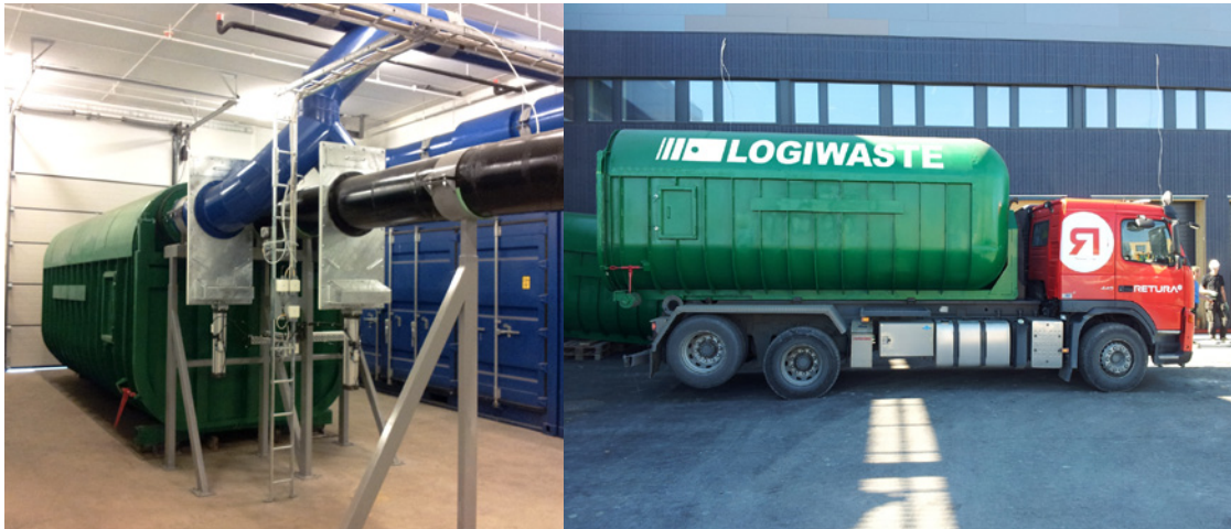
Above to left: Terminal building with container. Sorting at source is supported by each fraction of waste automatically being assigned to the right container.
