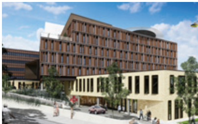
Regional hospital Viborg Hospital, chute Viborg, Denmark
