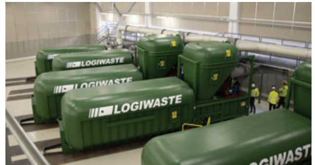
The terminal at Karolinska Hospital in Stockholm. Collection of four fractions of waste in filter containers and compactor containers.
