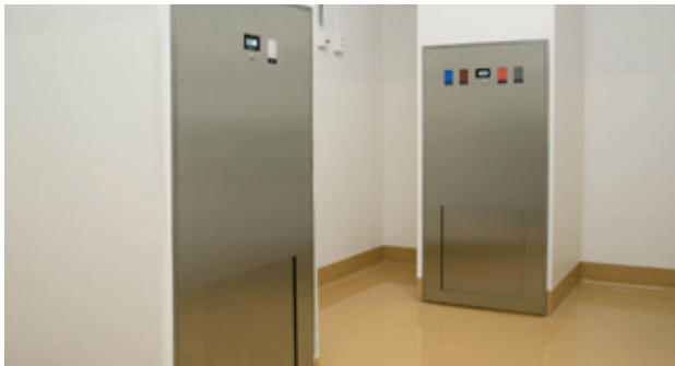
Fully automated, no-contact inlets make it easy, hygienic and comfortable for the personnel to introduce waste and laundry bags.
