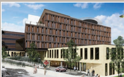
Regional hospital Viborg Hospital, chute system Viborg, Denmark
