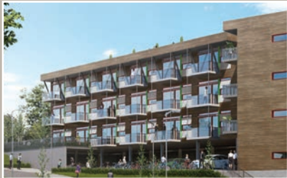
Tesliåsen Mobile waste vacuum system Trondheim, Norway
