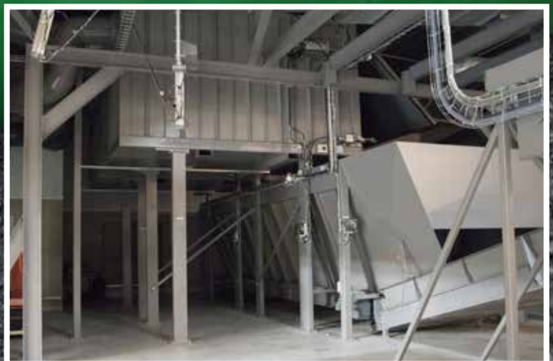
Picture on the right: System for handling laundry in the terminal at the Academic Hospital in Uppsala, where conveyor belt-fed laundry separators, load pockets and feed conveyors form a central part of the laundry management.
